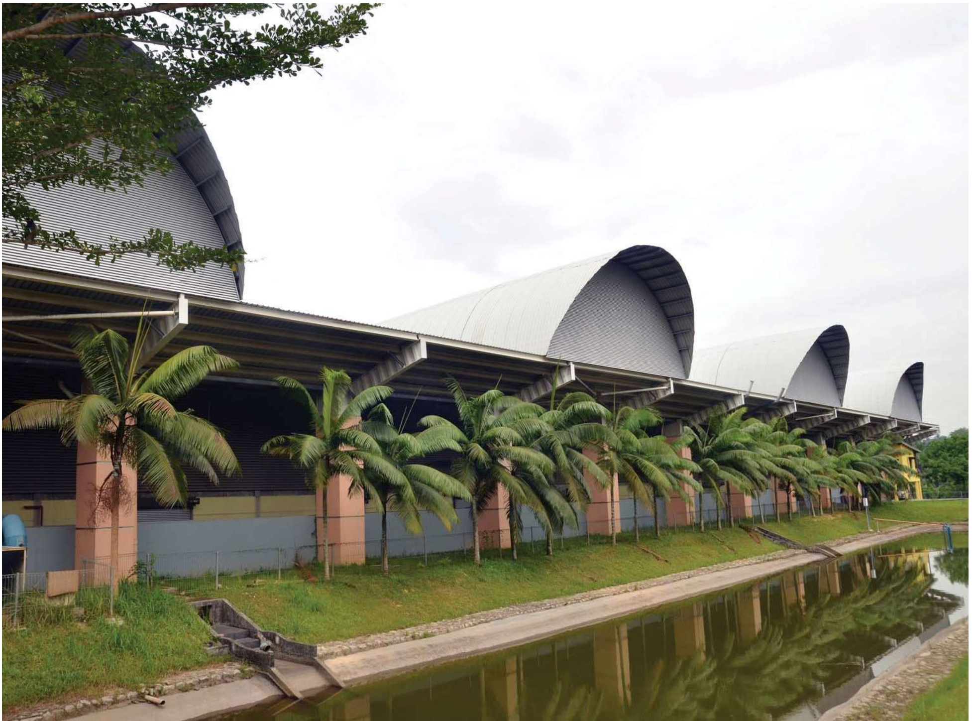
MHI aspires to become a sustainable and environmental friendly research laboratory. Shown here is the storage pond for rainwater harvesting which serve as one of the water sources for physical modelling.
