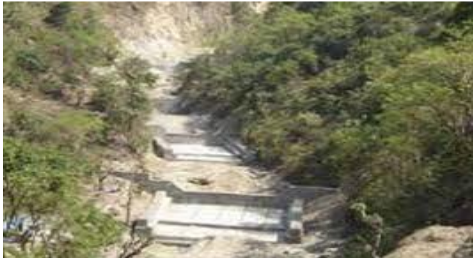
Sabo Dam in Khahare Khola
