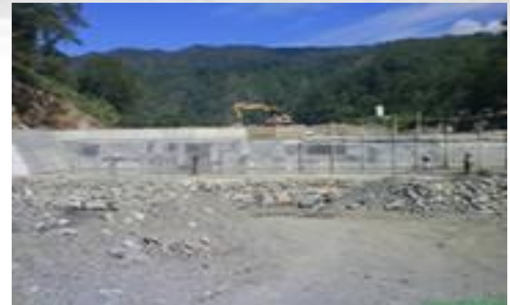
Sabo Dam Construction in May 2010
