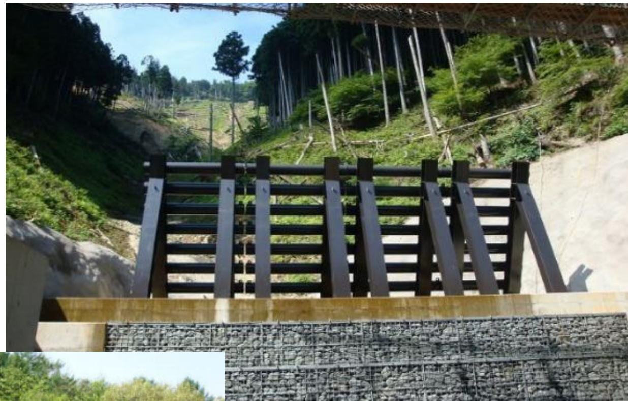
Open Sabo Dam at Nagai River, Japan
