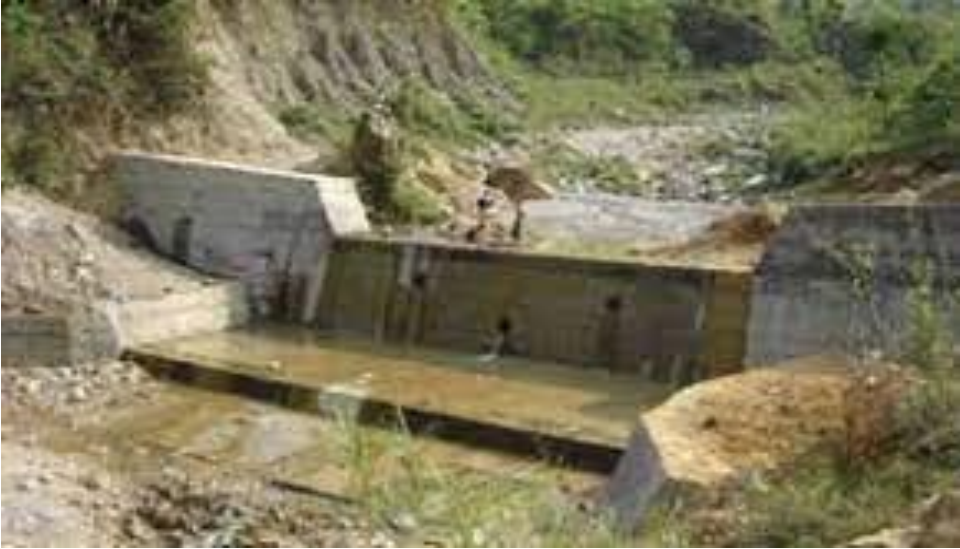
Sabo Dam in Ruwa Khola
