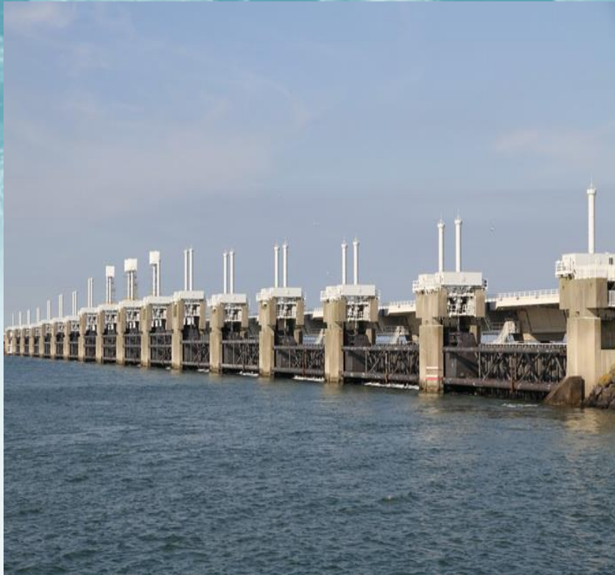
Flood Barrier - Netherland
