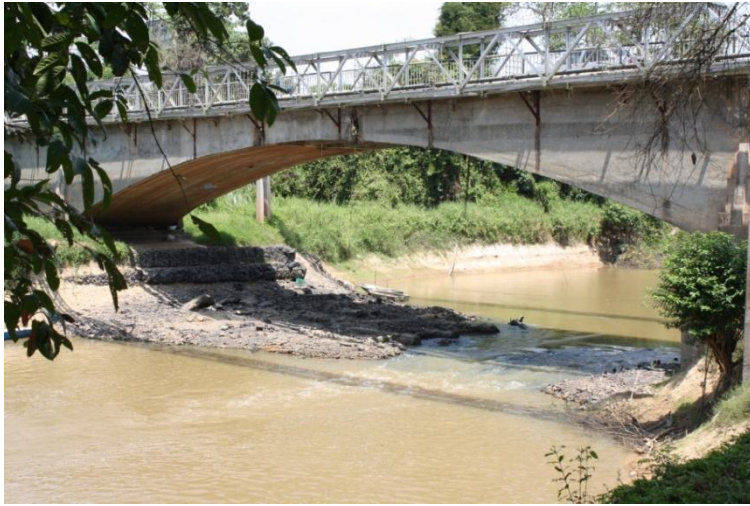
Sungai Muar bridge at Kg Tebing Tinggi (Segamat)
