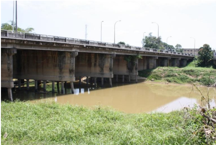
Sungai Muar bridge at Buloh Kasap (Segamat)
