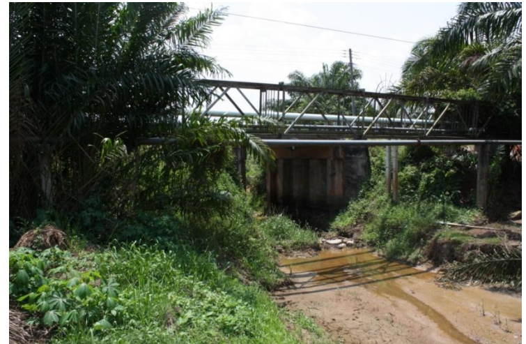
Sungai Ring bridge
