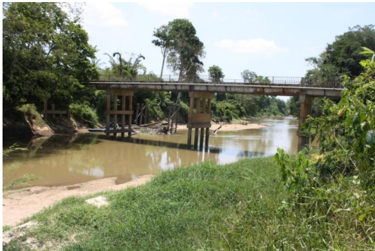
Sungai Muar bridge at Tumang (Segamat)
