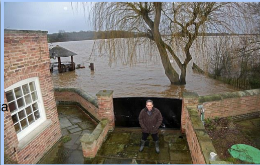
Brick floodwall, England
