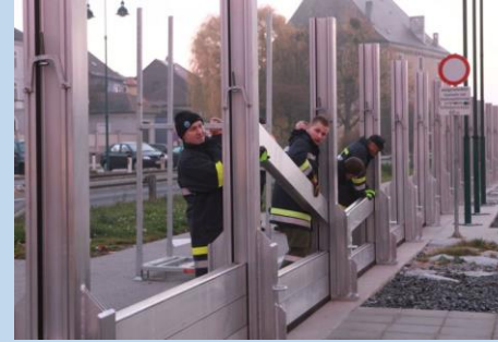
Mobile Floodwall, Austria
