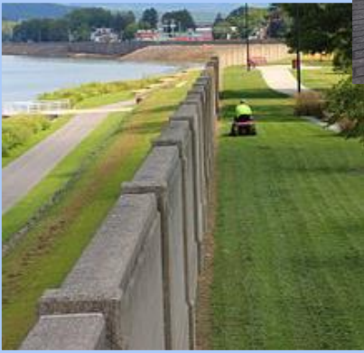
Floodwall in Sunbury, Pennsylvania
