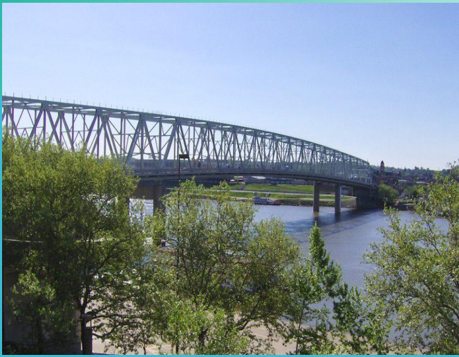
Taaylor-Southgate Bridge, Ohio and Kentucky, US-Truss Bridge
