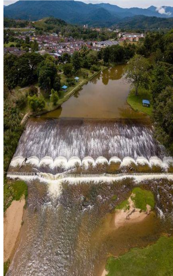
Image of Drone at Ampangan Pecah Source: Fb Hulu Selangor, 2024
