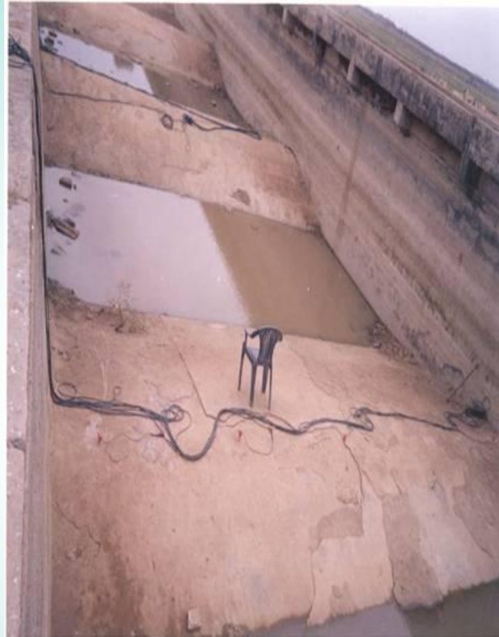
NDT by sonic transmission technique at Sardar Sarovar Dam, Gujarat, India.
