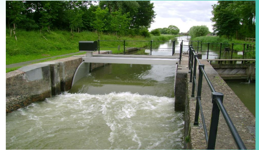
Tilt Gate Source: HC Waterbeheersing, 2024
