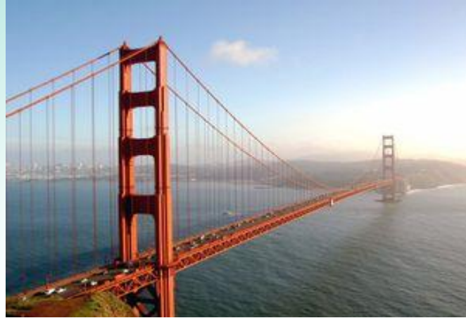
Golden Gate Bridge, San Francisco, US-Suspension Bridge
