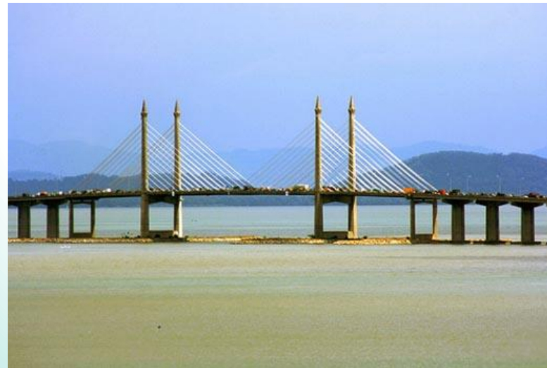
Penang Bridge, Malaysia- Cable-stayed Bridge
