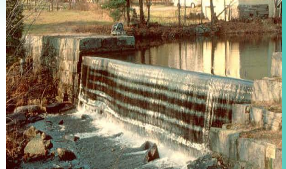
Broad-Crested Weir Sumber: HydroCAD, 2024
