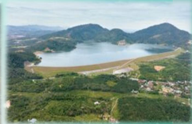
Storage Dam -Mengkuang Dam, Pulau Pinang Sumber: Kosmo, 2024
