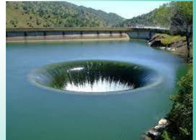
Morning Glory Spillway
