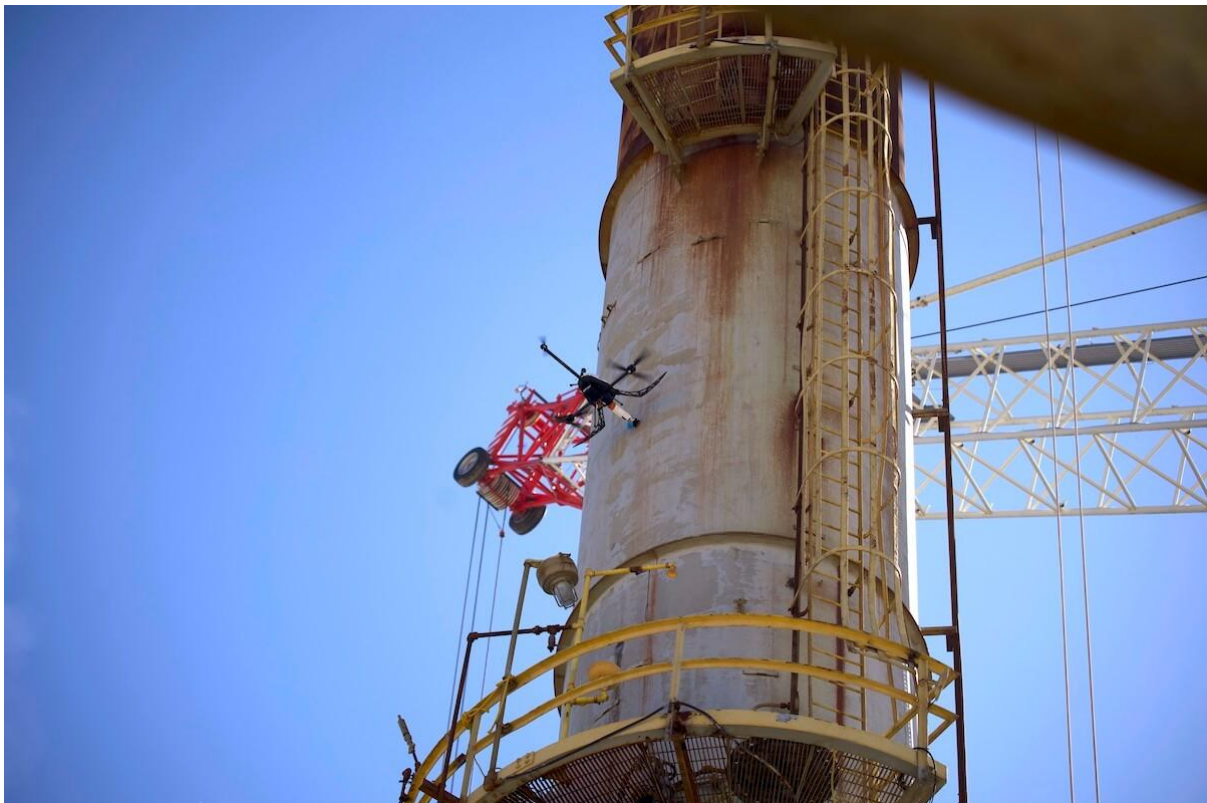
Figure 2. NDT by Visual Inspections using Drone at United States of America [10]
