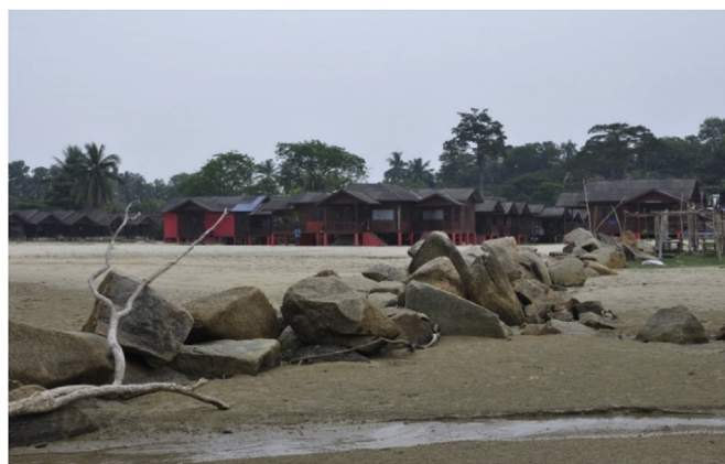
Fig. 7. Groyne protection structure on the Cherating beach.
