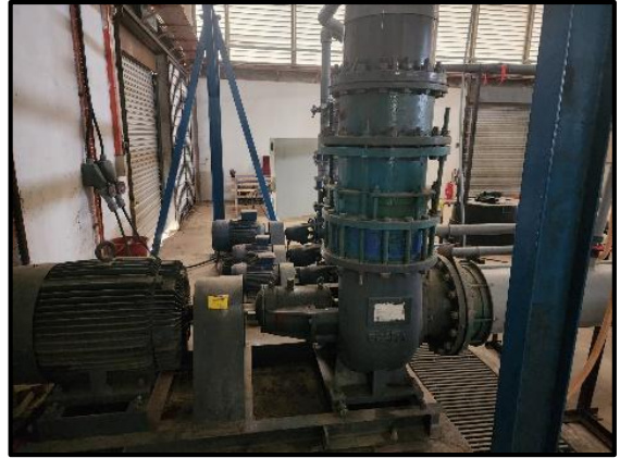
Figure 3: Ultrasonic Flow Meter and 50 HP water pump.
