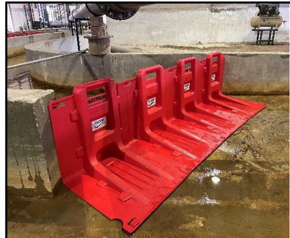
Figure 2: Installation of the Flood Control Baffle to contain and divert water
