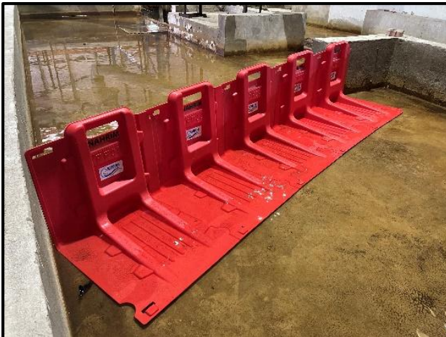
Figure 2: Installation of the Flood Control Baffle to contain and divert water
