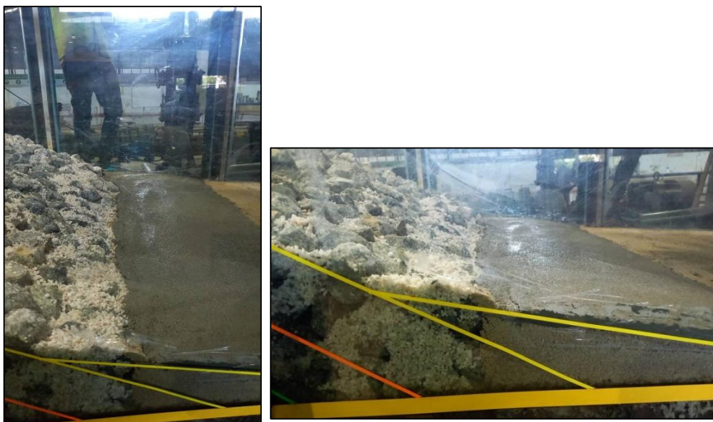
Figure 3.14: Cemented layer at toe of revetment base
