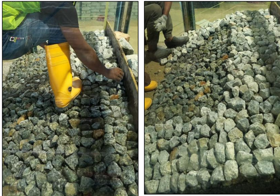
Figure 3.17: Laying of upper armour layer
