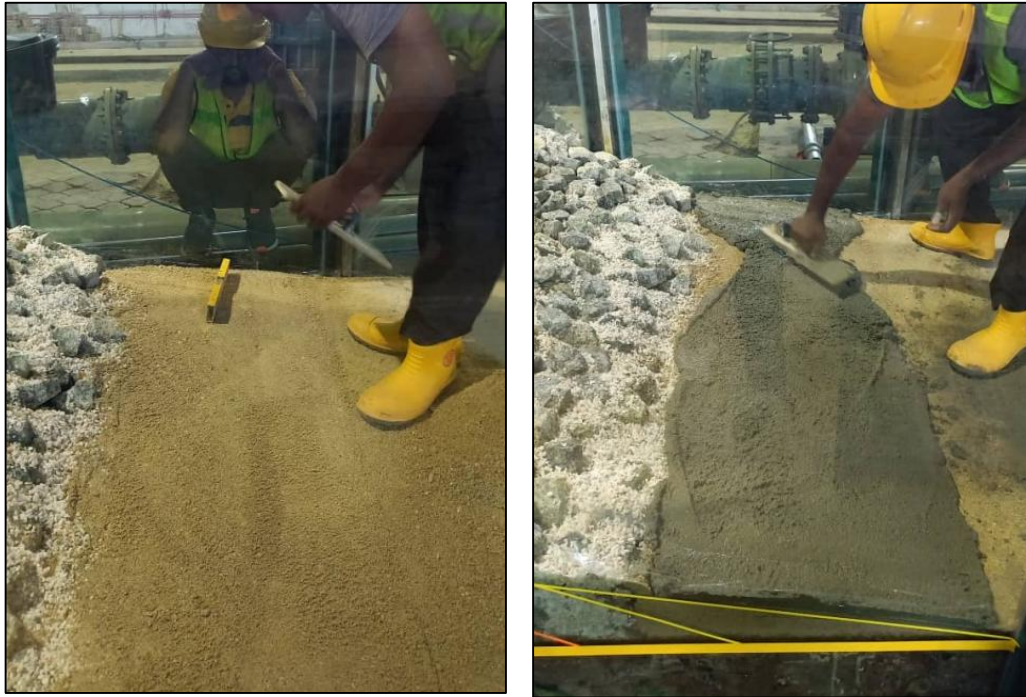
Figure 3.13: Rock revetment base layout
