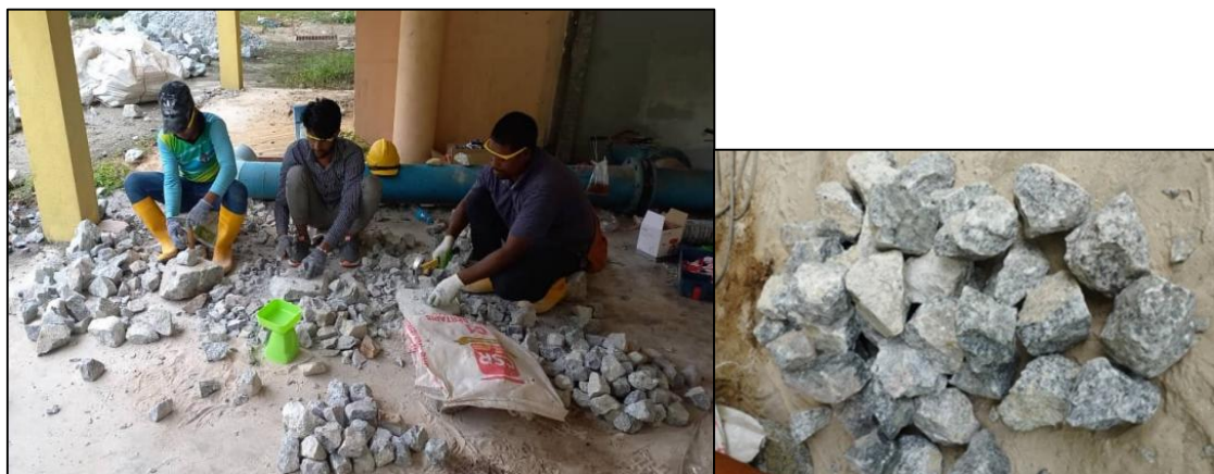
Figure 3.12: Breaking stones process according to pre-determined shape and weight for construction of rock revetment structure
