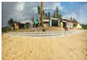
a. NEXC Block installation in Marang, Terengganu
