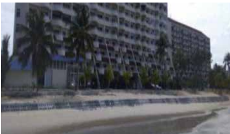
b. NEXC Block structure in Port Dickson, Negeri Sembilan
