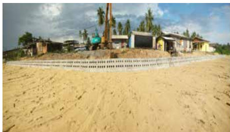
a. NEXC Block installation in Marang, Terengganu
