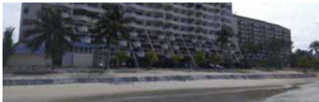
b. NEXC Block structure in Port Dickson, Negeri Sembilan
