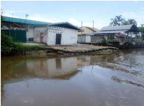
Figure 61: The roads were destroyed and vulnerable to fuel pump stations near to river banks
