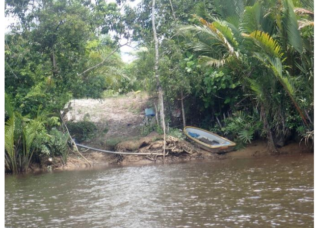
Figure 35: High erosion of river bank and produced flood prone areas
