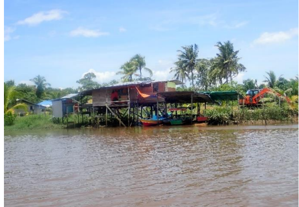
Figure 64: Local residents house near the river bank
