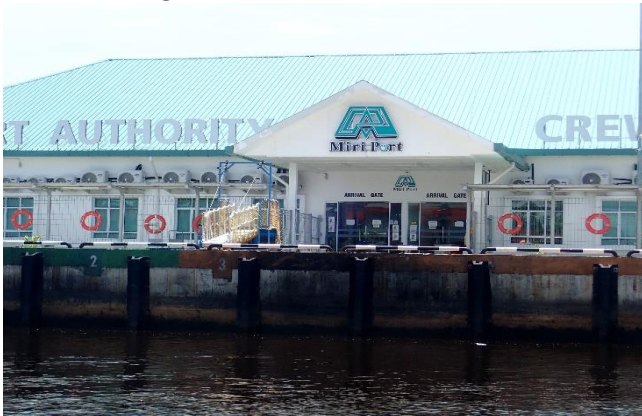
Figure 98: the headquarter of port authority
