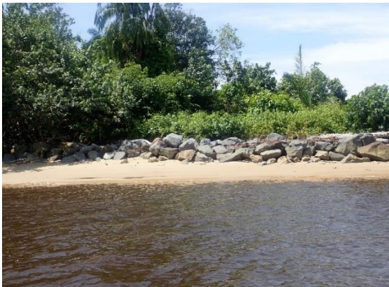
Figure 73: The hard structures were build as revetment to protect river estuary
