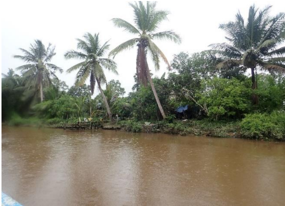
Figure 51: The moderate erosion of river banks adjacent to local residents house
