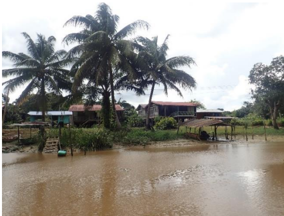
Figure 49: The small jetty for local residents.
