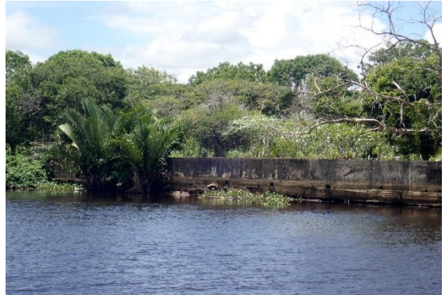
Figure 95: The river bank structue as revetment to protect river bank erosion
