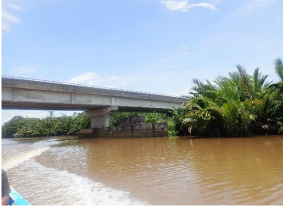
Figure 63: The bridge to connected two villages
