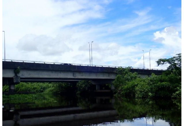
Figure 91: The bridge to connected two villages
