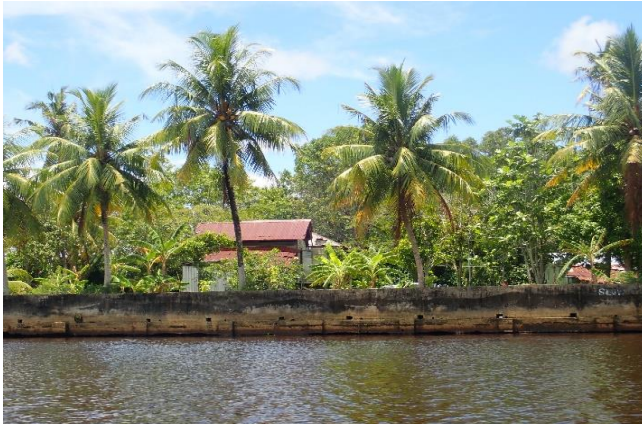
Figure 94: The river bank structue as revetment to protect river bank erosion
