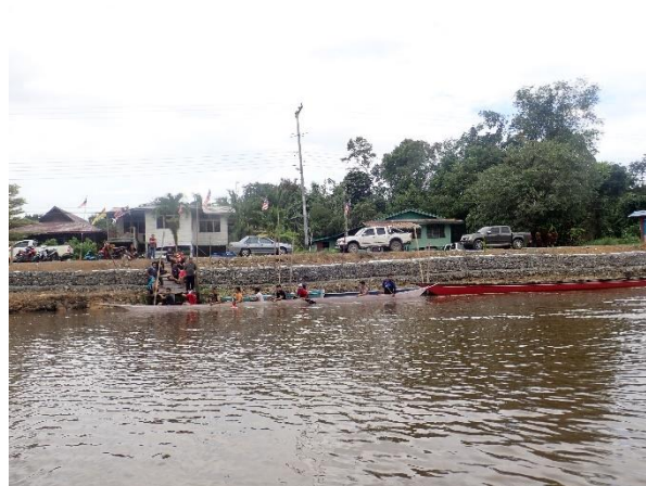
Figure 3: Some revetments were builded to protect Niah's River Bank
