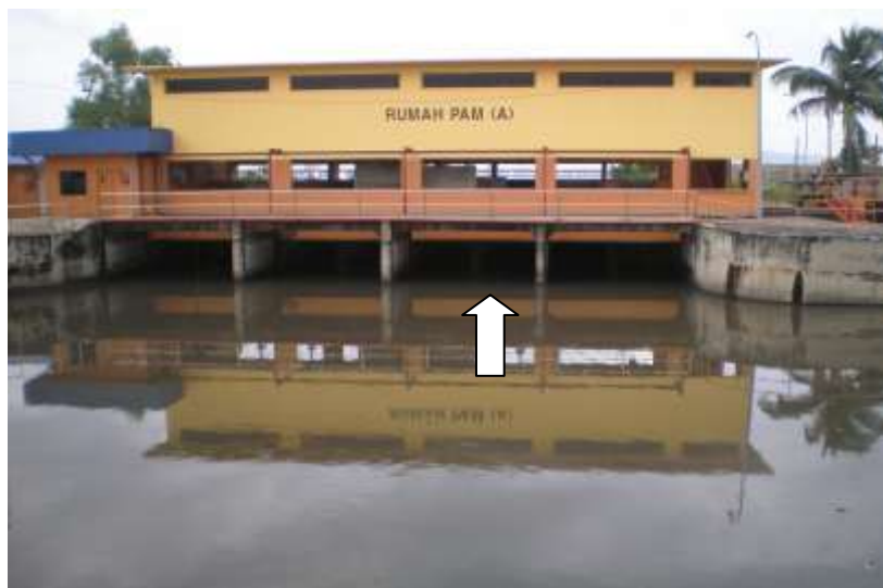
Fig 1. Inlet of a Pump A house.
