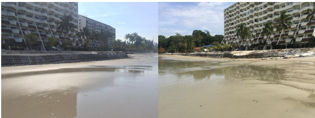
Figure 4.67 : Test site on 14 October 2016, a few blocks of the product settled due to scouring of old piping structure underneath. Severe erosion problem occurred at the end of the product alignment and afterwards (source : NAHRIM)
