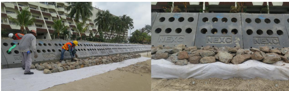
Figure 3.38 : Armour rock is stacked nicely to form a layer of mini revetment system for the NEXC blocks structure (source : NAHRIM)
