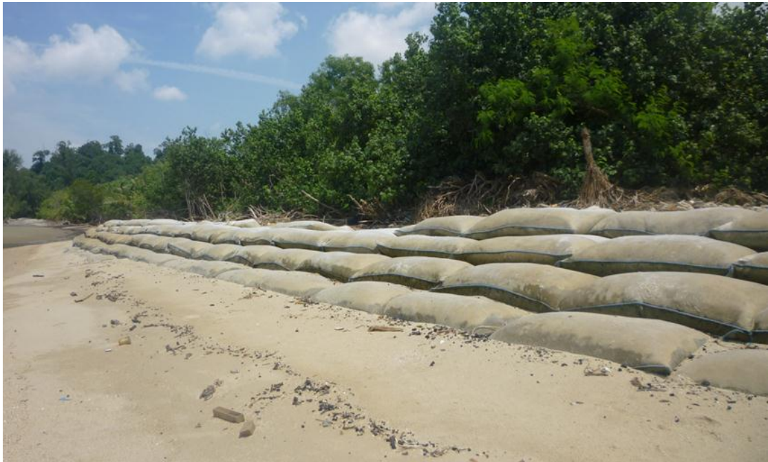
Figure 2.35 : Sand bags at Pantai Penggorak, Kuantan (source : DID, 2009)
