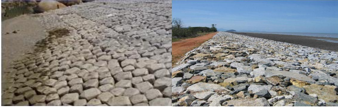
Figure 2.13 : Basalt revetment in Melaka (left) and quarry stone revetment in Kedah (right) (source : DID, 2009)
