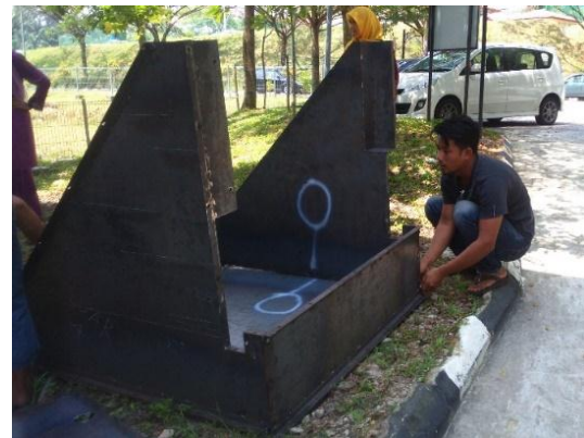
Figure 3.24 : The Fabrication of Mould's framework for NEXC Block (source : NAHRIM)
