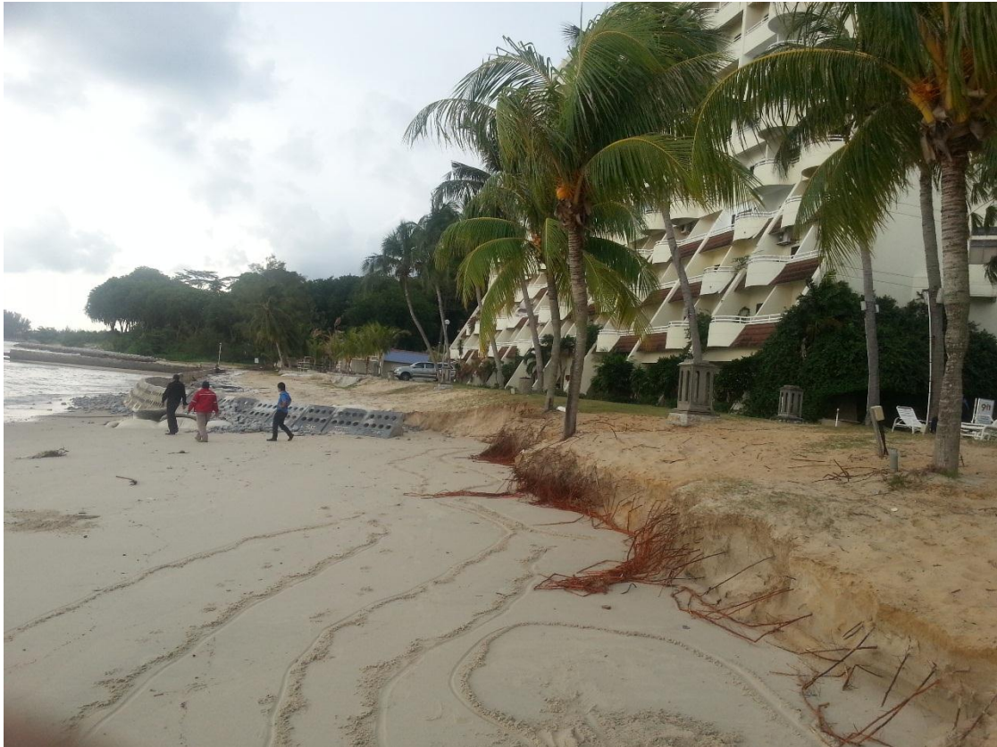
Figure 3.41 : Severe erosion occurred at the end of the chainage 108m of NEXC Blocks System and afterwards after the Southwest Monsoon season (source : NAHRIM)
