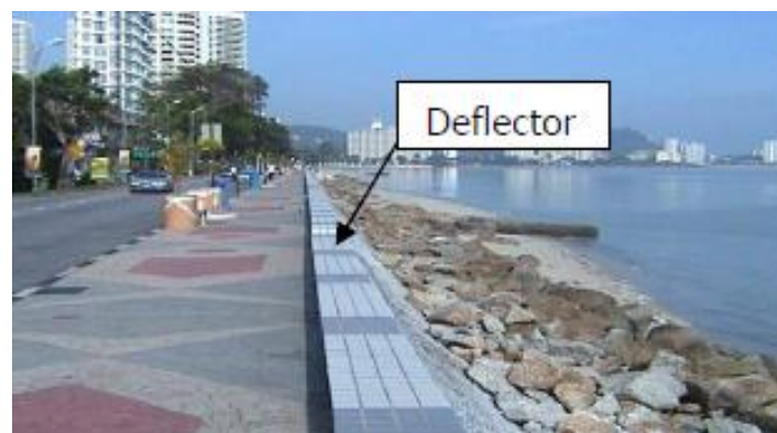
Figure 2.31 : Seawall with run-up deflector made to blend as part of the landscape at Gurney Drive, Penang (source : DID, 2009)
