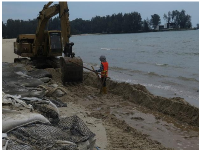
Figure 3.32 : Excavation and levelling works at test site (source : NAHRIM)
