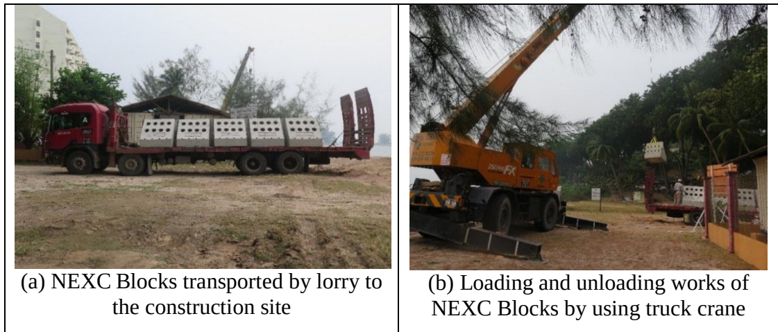
Figure 3.34 : Transportation and Handling of NEXC Blocks to Construction Sites (source : NAHRIM)
