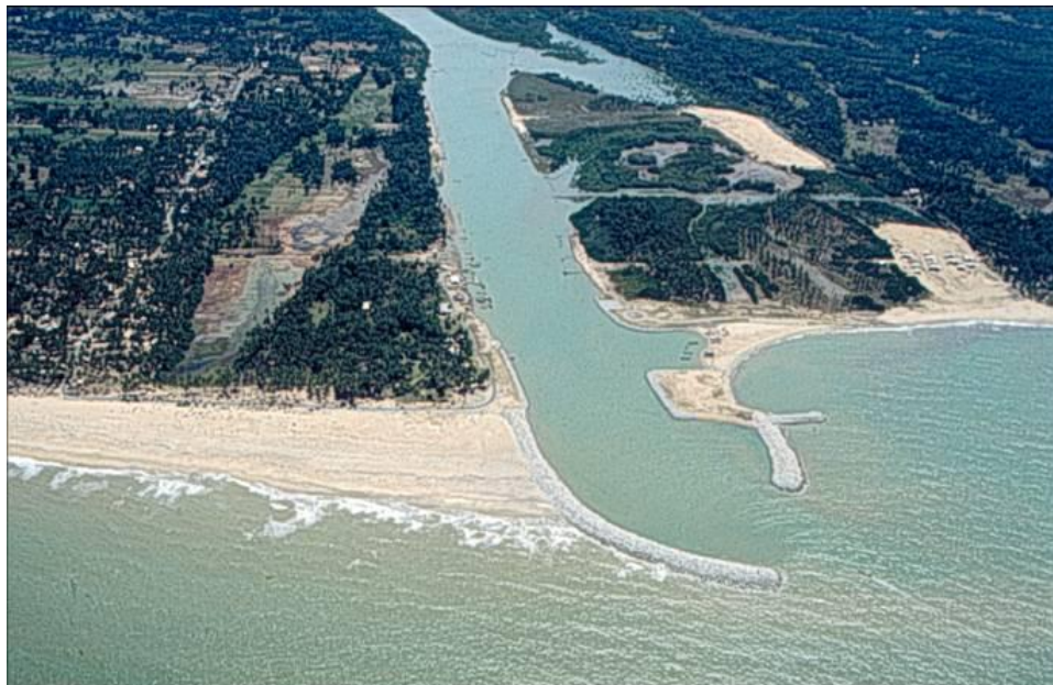
Figure 2.22 : Breakwaters at Sungai Marang river mouth, Terengganu (Source : DID, 2009)
