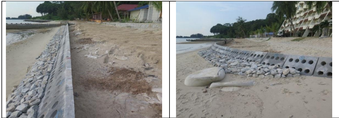
Figure 3.40 : The view on the test project site after the completion of site finishing works (source : NAHRIM)
