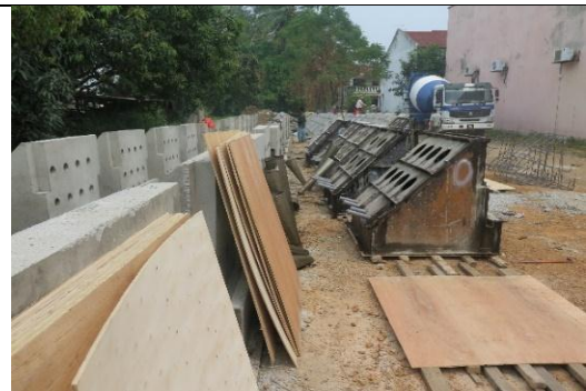
(b) Steel plates and plywood are used in the installation works
