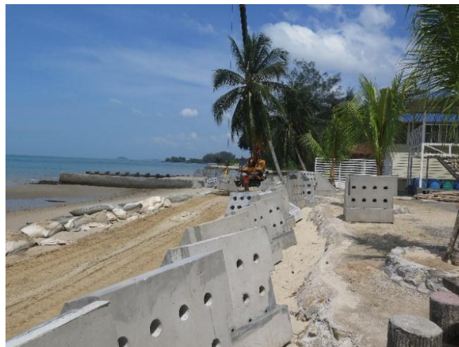
Figure 3.35 : Site Preparation and Clearing for the Construction Project of NEXC Blocks System (source : NAHRIM)
