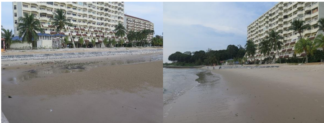
Figure 4.65 : Test site on 21 November 2015, additional scour protection at toe (source : NAHRIM)
