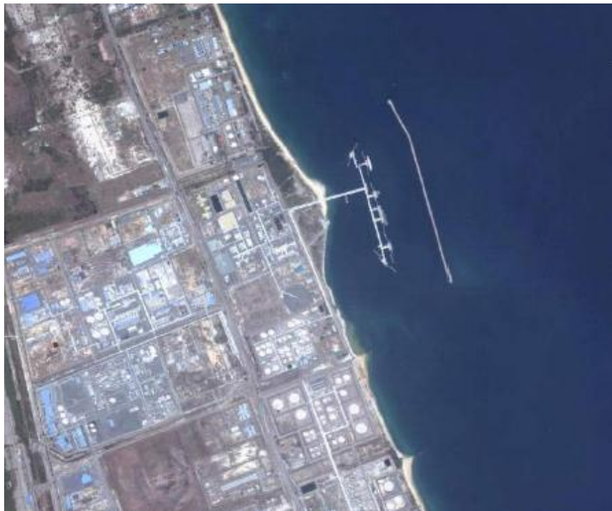
Figure 2.23 : Offshore breakwater at Kertih, Terengganu (source : DID, 2009)
