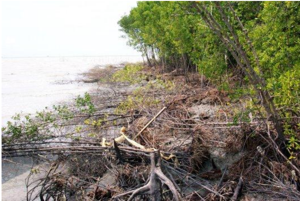
Figure 2.6 : The mangrove erosion in Tanjung Piai wrought by wave action brought on by increased shipping traffic due to the function of a new international sea port nearby. (Source : http://ramsar.rgis.ch/cda/en/ramsar-news-archives-2003-ramsar-visit-to-new/main/ramsar/1-26-45-86%5E16294_4000_0__ )
