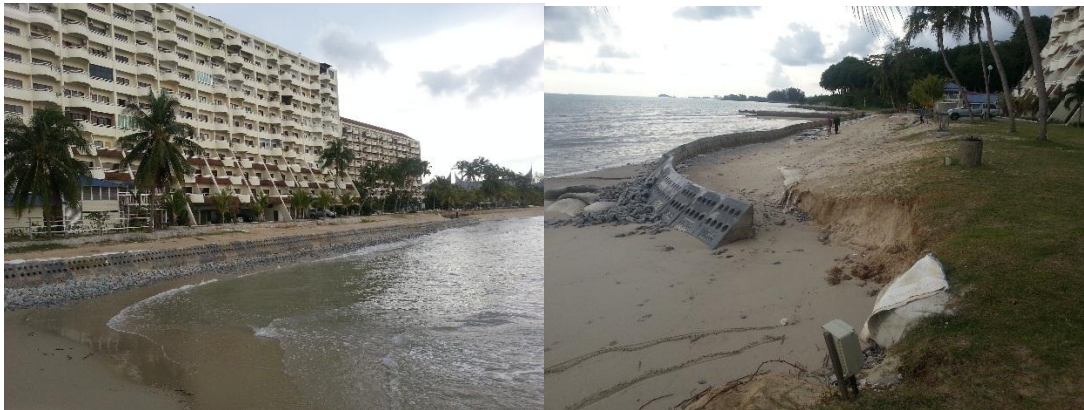
Figure 4.66 : Test site on 20 July 2016, erosion problem occurred at the end of the product alignment (source : NAHRIM)
