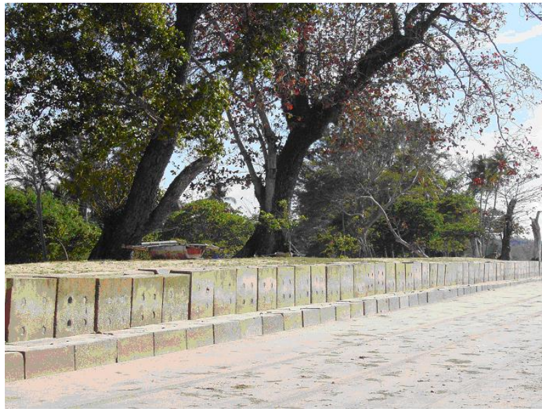
Figure 2.26 : First generation Labuan Blocks as vertical cubic blocks-Pancur Hitam, Wilayah Persekutuan Labuan (source : DID, 2009)
