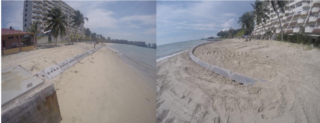
Figure 4.64 : Test site on 6 November 2015, post construction (source : NAHRIM)
