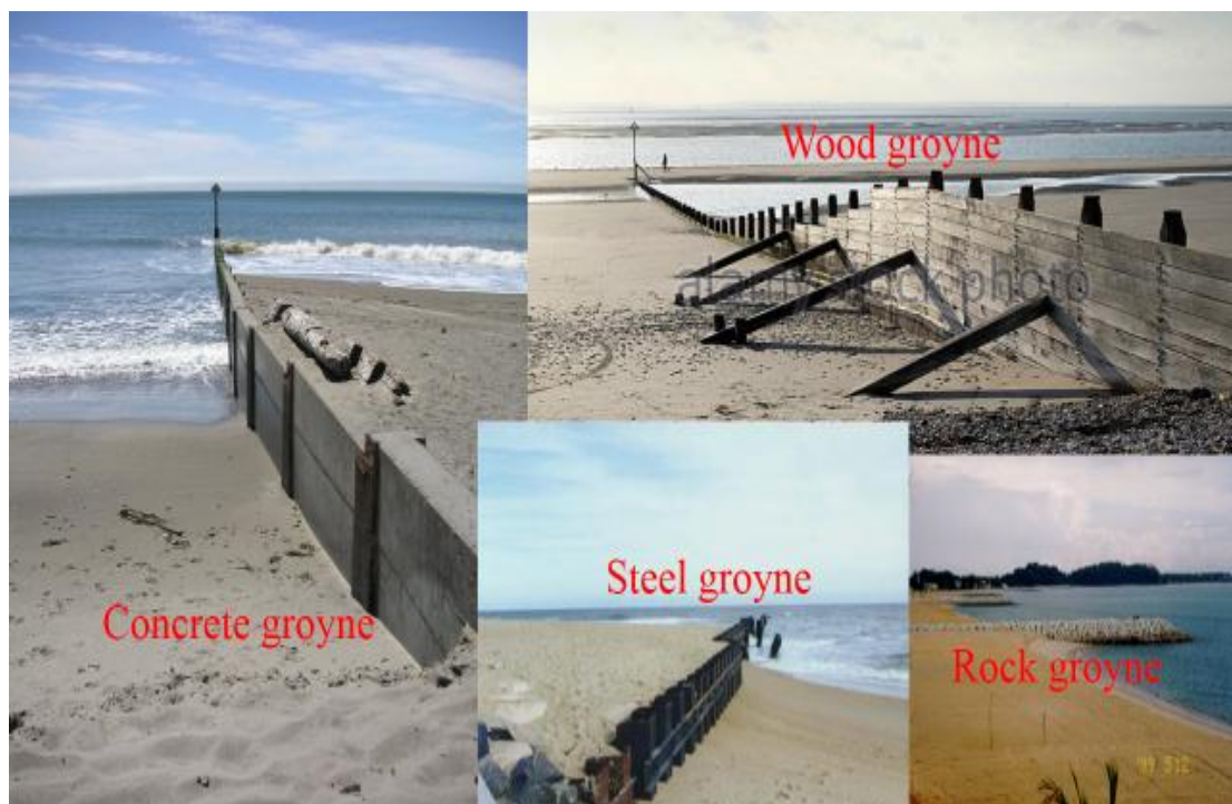
Figure 2.17 : Various types of groynes materials (source : internet)
