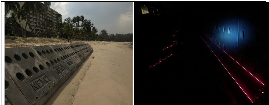
Figure 3.39 : Straight Fine Tune Alignment of NEXC Blocks Structure on Test Site (source : NAHRIM)
