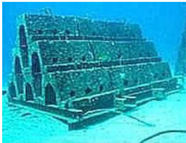
Figure 2.25 : Submerged 3-layered WABCORE breakwater and artificial reef with narrow crest arrangement at Panuba Bay, Tioman Island, Pahang (source : Mohd, 2013)
