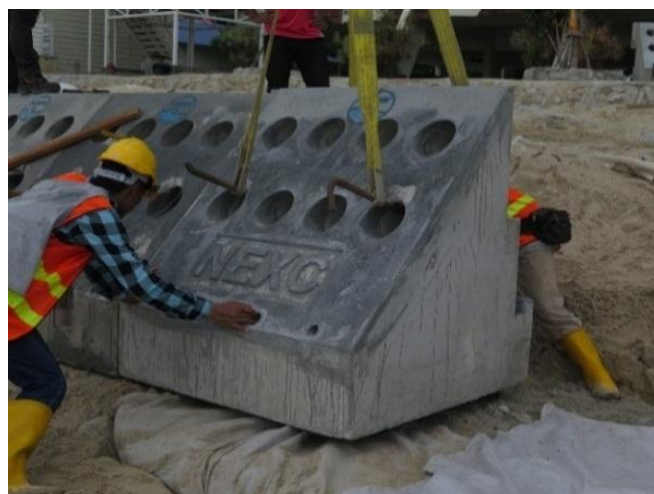
Figure 3.36 : Lifting of NEXC Block on Site by Using Safety Cable (source : NAHRIM)
