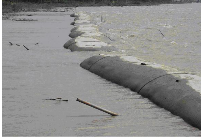
Figure 2.34 : Geotube at Tanjung Piai, Pontian, Johor (source : DID, 2009)
