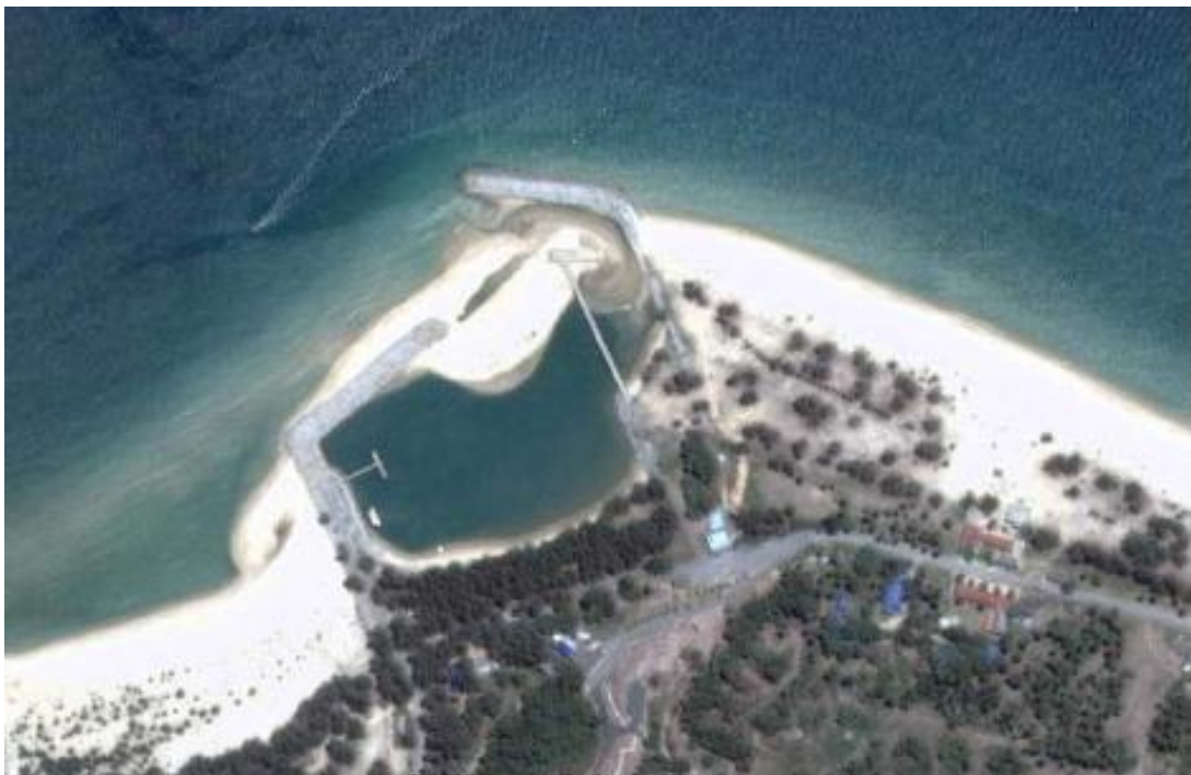
Figure 2.24 : Deposition of sediment in front of Merang Breakwaters and jetty (source : DID, 2009)
