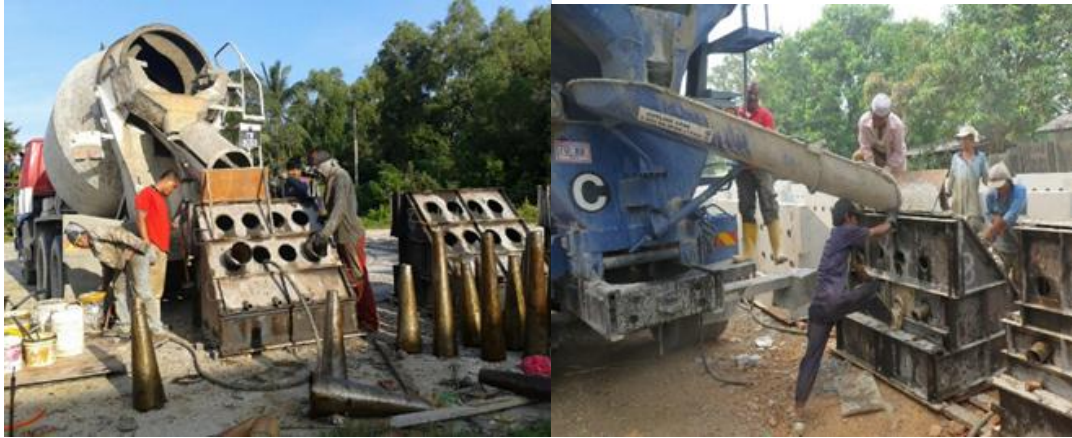
Figure 3.26 : Concrete Casting Works at Site (source : NAHRIM)
