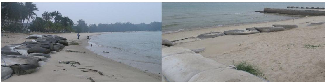
Figure 3.22 : The Placement of Sandbags System to Prevent Erosion on The Beach (source : NAHRIM)
