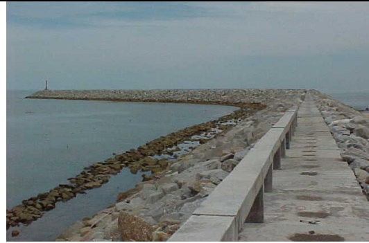
(f) shore connected breakwater
