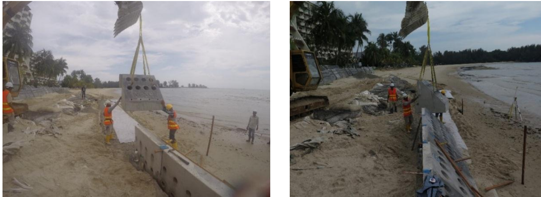
Figure 3.37 : The deployment of the NEXC Blocks System on test Site (source : NAHRIM)
