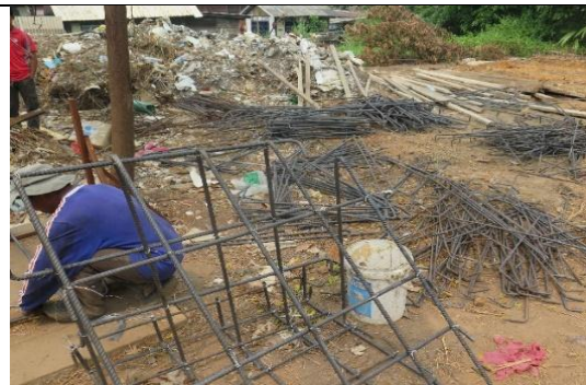
(a) Steel bar that used as a reinforcement
