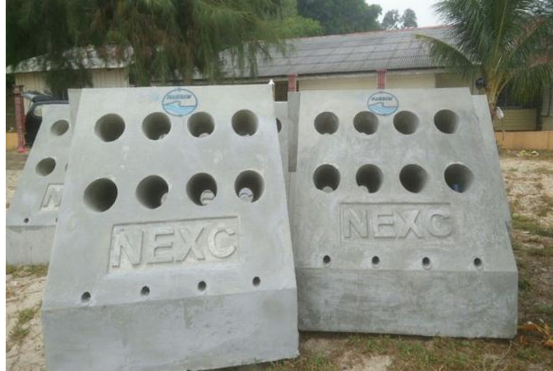
Figure 3.4 : The holes on the NEXC block unit (source : NAHRIM)
