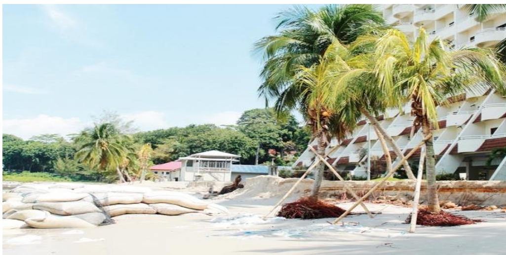
Figure 1.7 : Coastal erosion problem just behind the building of Regency Hotel, Tanjung Tuan, Batu 5, Port Dickson (source : Sinar Harian, 2013)
