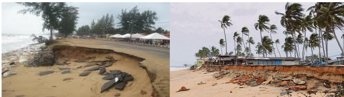
Figure 2.5 : Coastal erosion at Pantai Tok Jembal (left) and Pantai Kampung Tanjung Gelam (right), Mengabang Telipot, Kuala Terengganu, Terengganu (source : https://ainanatasha94.wordpress.com/2014/11/11/hakisan-pantai-tok-jembal/ and http://www.hmetro.com.my/node/104335 )
