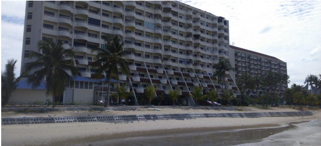
Figure 3.3 : NEXC Block System at Pantai Batu 5, Port Dickson (source : NAHRIM)
