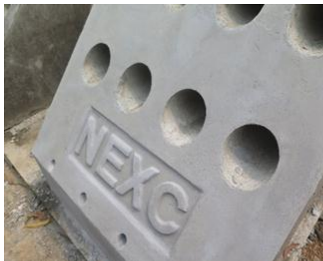
Figure 3.28 : Final Touch-up of NEXC Block Surface (source : NAHRIM)
