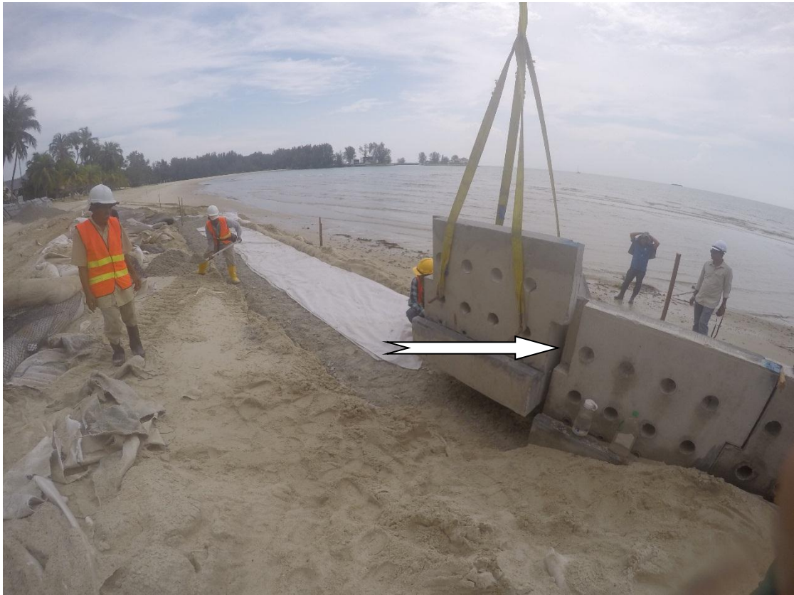
Figure 3.9 : The arrow shows slotted (male connector) and grooved (female connector) interlocking designed for NEXC Blocks System (source : NAHRIM)
