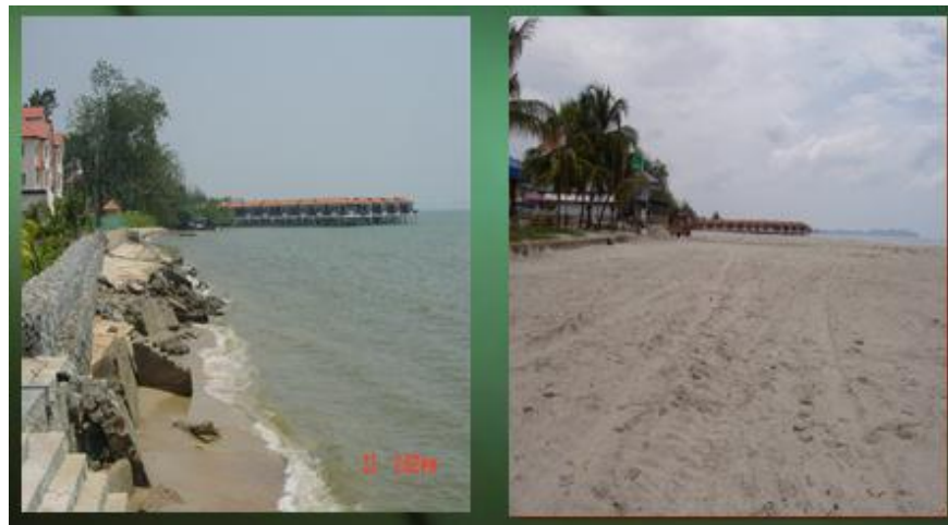
Figure 2.32 : Beach nourishment project in Port Dickson. Left figure is the view of shoreline before the project started while the right figure shown that the view of the new beach formed just after the project completed. (source : DID, 2009)
