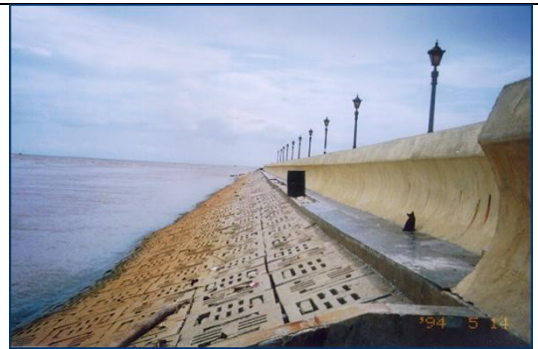
(b) Interlocking flex-slab revetment and Seawall structures
