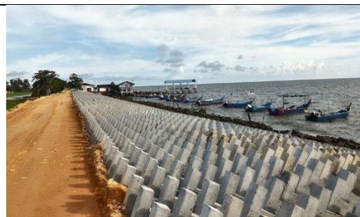
(c) Earth bund and sauh revetment
