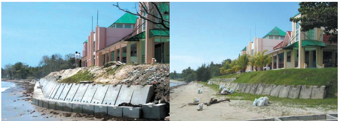
Figure 2.29 : Initial beach condition in year 2000 (left) and stabilized beach condition in year 2005 (right) after placement of Labuan Blocks as a coastal protection control measures at Kiamsam Beach, Wilayah Persekutuan Labuan (source : Jurutera Bulletin April 2006, BEM)
