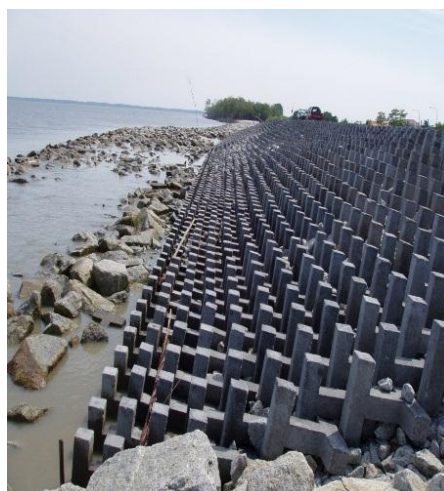
Figure 2.16 : SAUH Revetment that was constructed in Selangor Coastline (source : DID, 2009)
