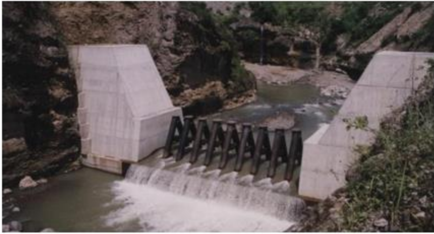
Figure 1: Open Sabo Dam in Indonesia
