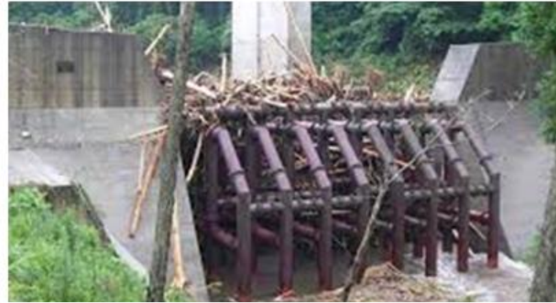
Figure 2: Open Sabo Dam (Kitazato River dam) in Japan
