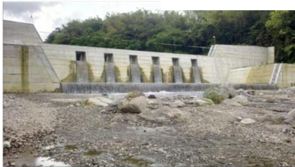
Figure 3: Open Sabo Dam in Kabupaten Magelang, Middle Java, Indonesia
